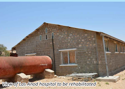
View of Sanaag regional hospital to be rehabilitated
