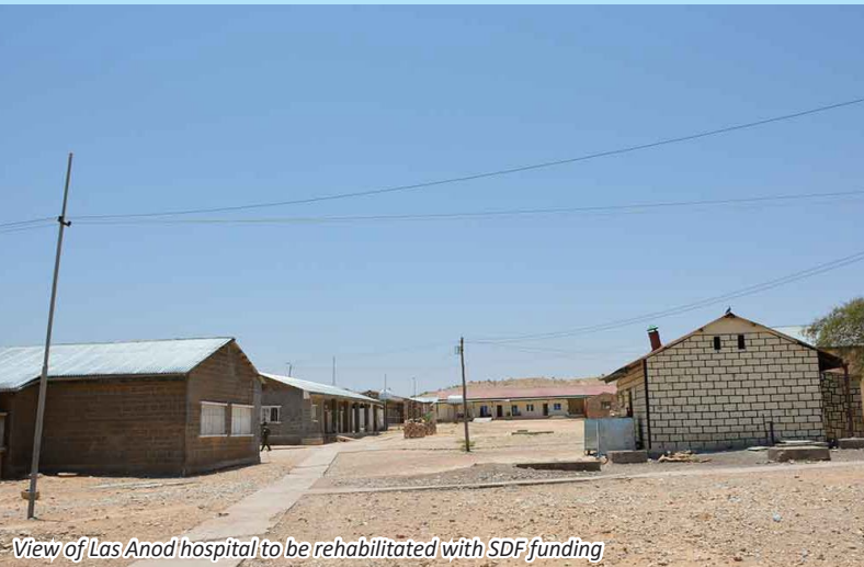
View of Las Anod hospital to be rehabilitated
